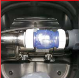
Check valve and sewage pump
